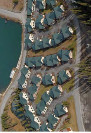
Cool colored metal roofs. Photo: Custom Bit Metals
