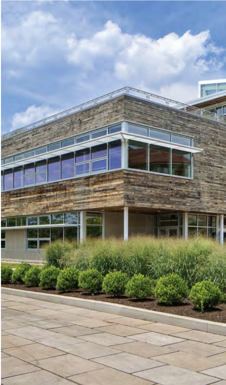
Center for Sustainable Landscapes The Design Alliance Architects Pittsburgh, Pennsylvania, United States Credit: Denmark Photography, Inc.
