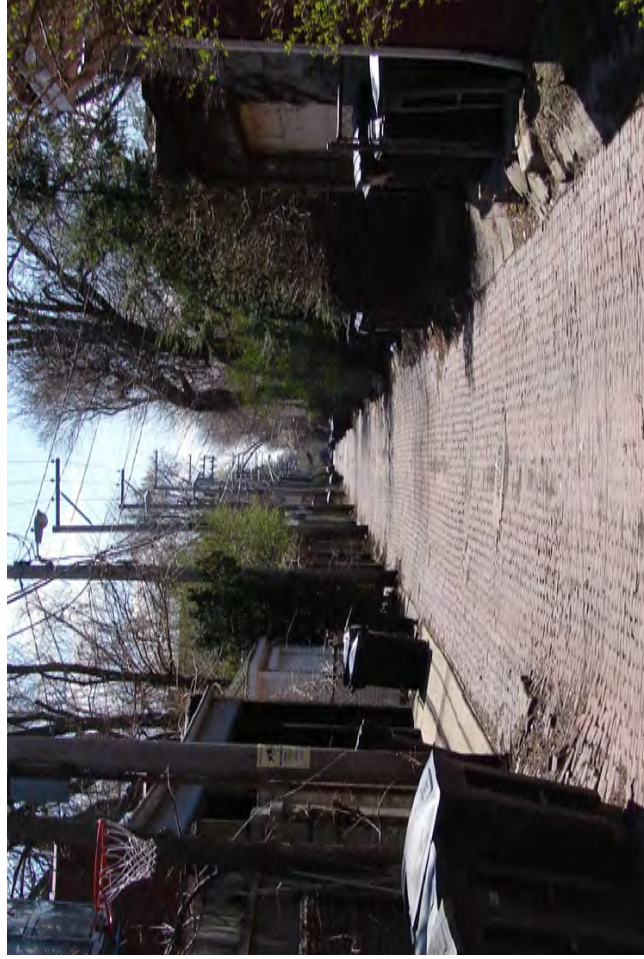
In Chicago there are 1,900 miles of alleyways, only part of the total 3,500 acres of impermeable surfaces in the city. Photo: City of Chicago
