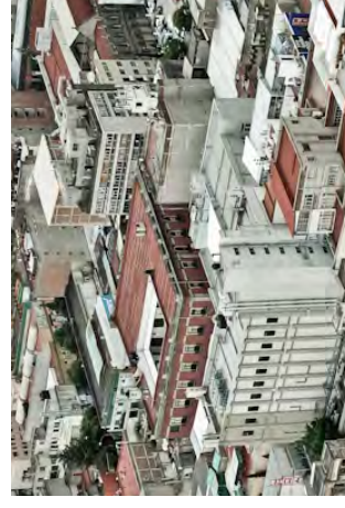
Urban rooftops in Mexico City. Photo: Storkholm Photography
